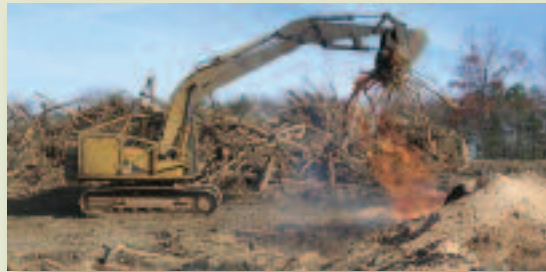
Stumps and debris are pit burned where permitted or ground up where burn permits are not obtainable.
