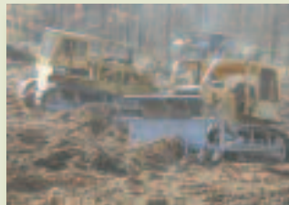
Stumps and debris are pit burned where permitted or ground up where burn permits are not obtainable.
